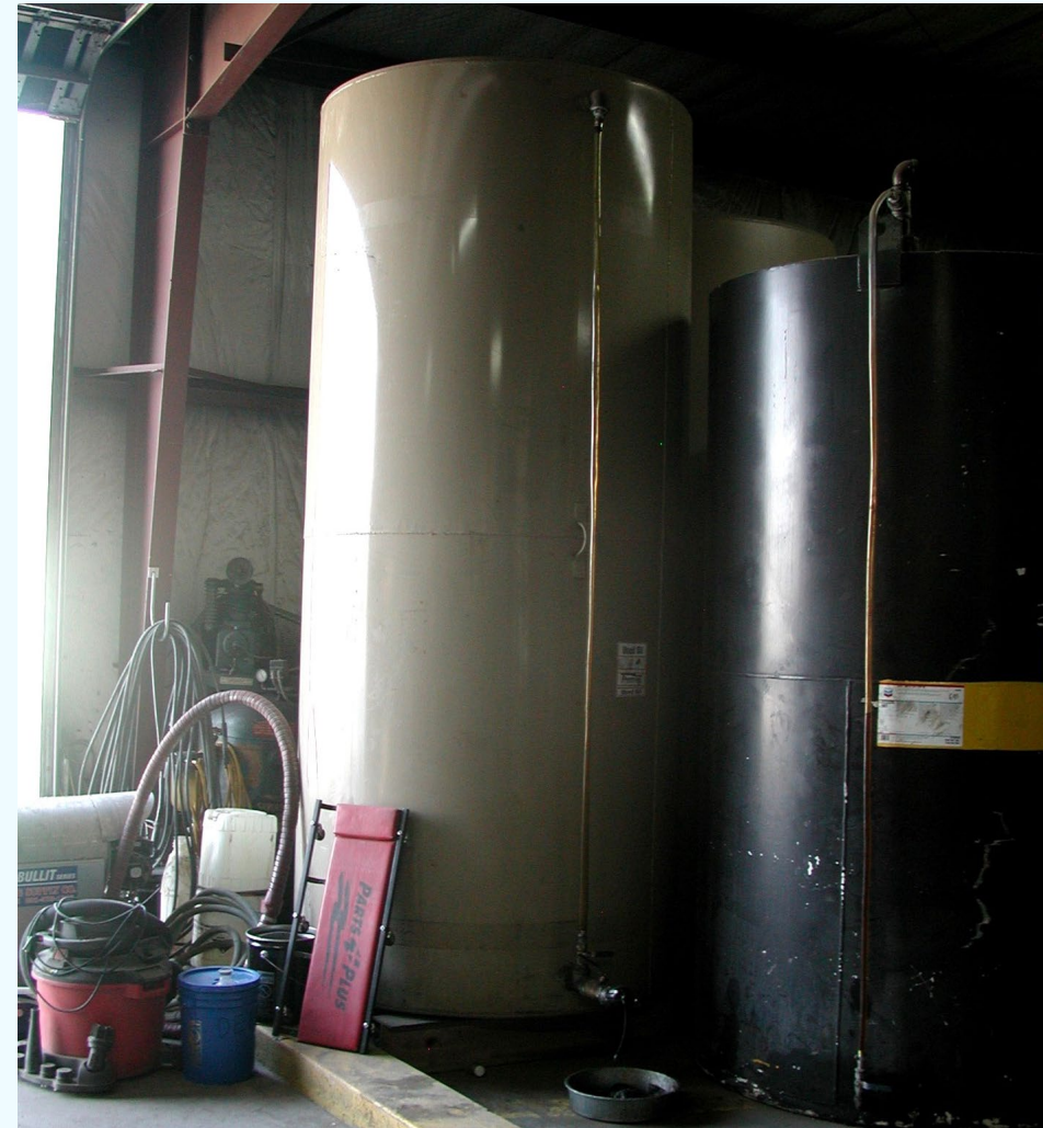
Tank in good condition (though crowded).
